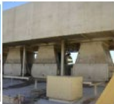
Prevent entry into the house
